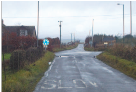
Photo 3.6.2: Mini-roundabout on national speed limit road – at this site the approach roads are narrow country lanes where the speeds are constrained.
