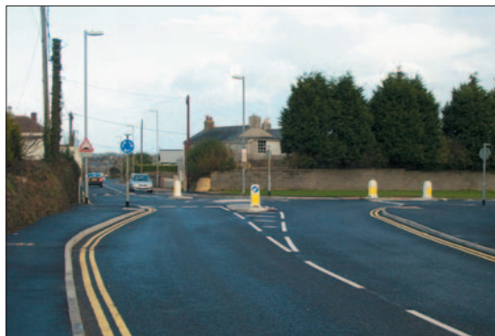
Photo 4.2.4: Deflection through alignment and traffic island
