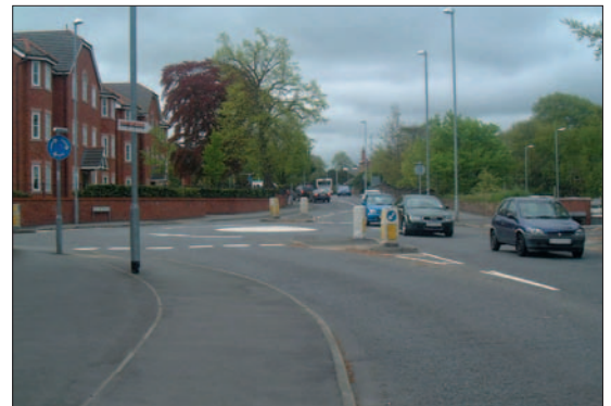
Photo 4.2.6: Approach deflection through alignment and traffic islands
