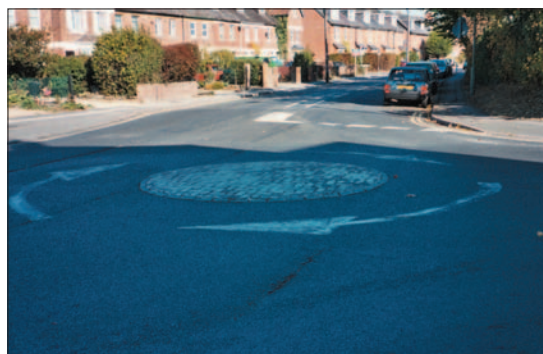
Photo 4.5.2: White paint wearing on blockwork central island
